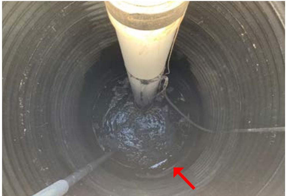
Figure 6. This submersible pump at the NDSU Langdon Research Extension Center tiled research site is not pumping water despite standing water at a low spot on Sept. 13, 2019, due to the poor soil water infiltration resulting in reduced drainage performance. The main drain is indicated by the arrow. (N. Kalwar, NDSU)
